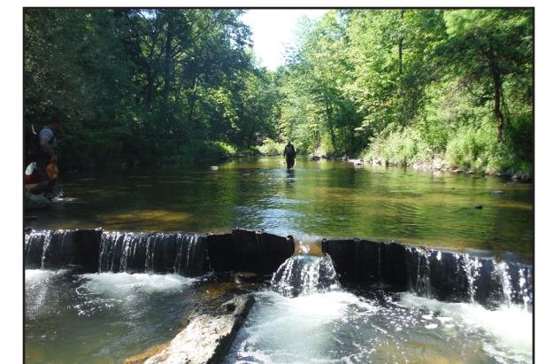
Example of a Fish Barrier Limiting Fish Passage - East Branch Cazenovia Creek
